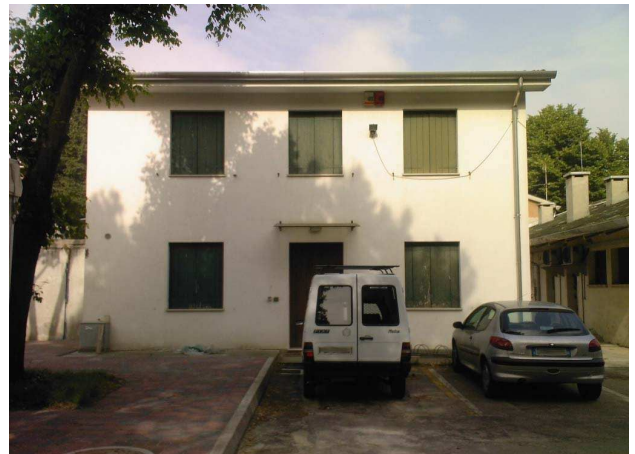
Fig. 2. Front face of the building.
